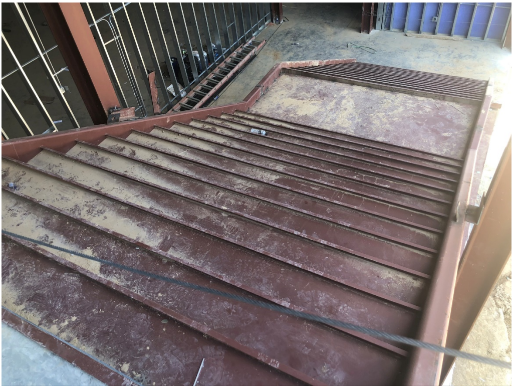
Figure 10 – 2 nd Level Stair at West Structure
