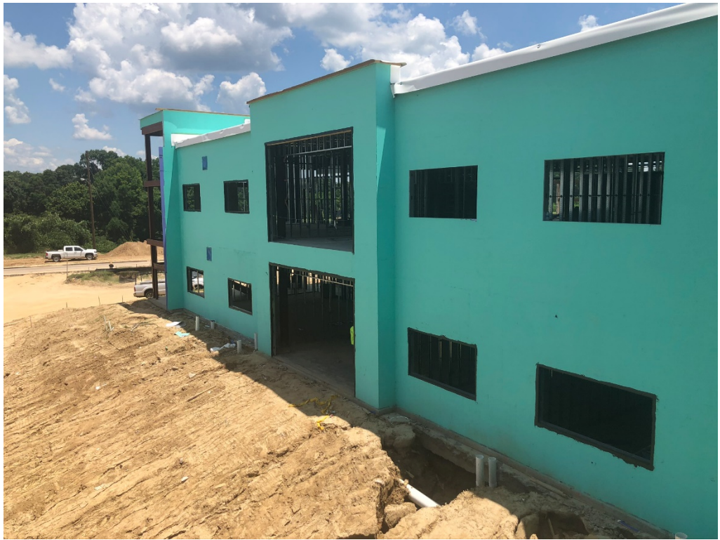
Figure 13 – West Elevation at North Structure
