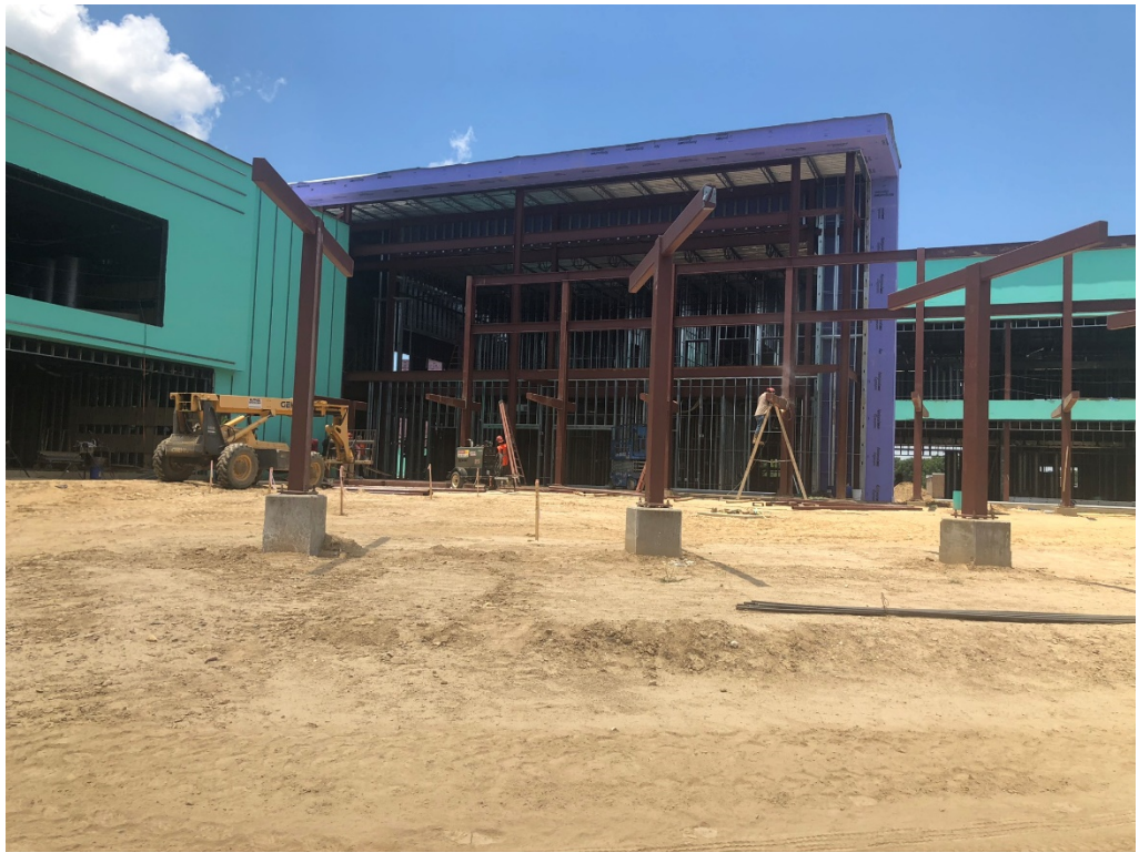
Figure 15 – Structural Steel Welding @ East Façade of North Structure
