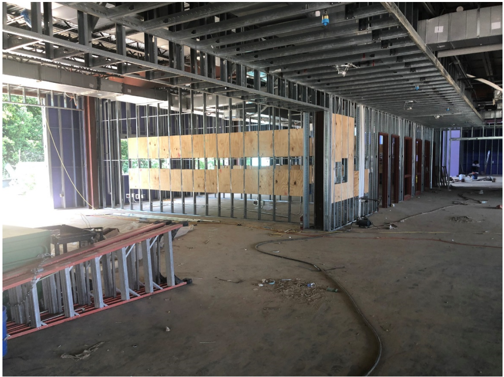
Figure 3 – Blocking in East Structure Ongoing
