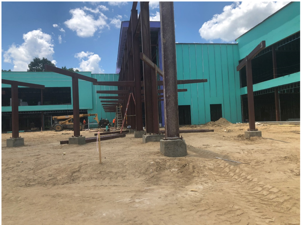
Figure 16 – Structural Steel Welding @ East Façade of North Structure
