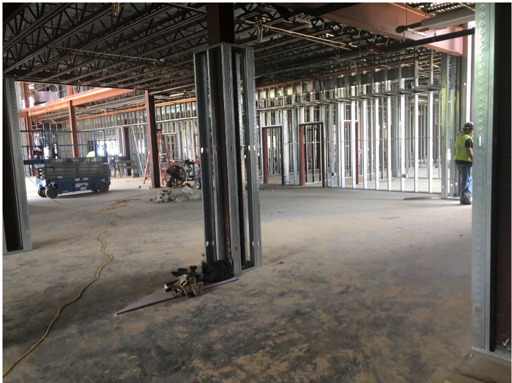
Figure 4 –Interior Framing Ongoing
