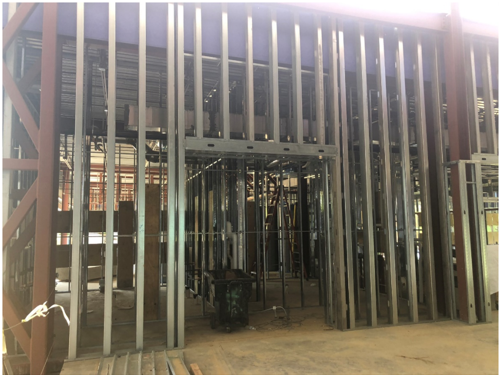
Figure 14 – Secondary Structural Wall Installed Between Central and East Structures
